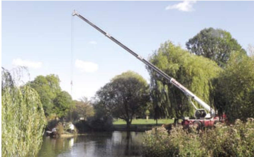
The hundred foot crane gets to work
