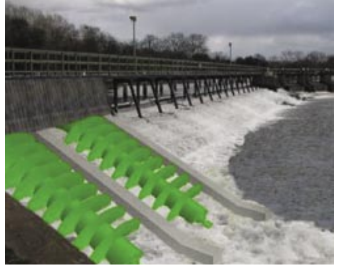
An indicative representation of the turbines – we plan to install 4 Archimedean screw turbines on a different section of the weir
