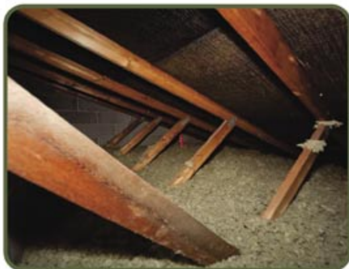
One household recently had loft insulation installed and is now in the process of having solar photovoltaic panels fitted to their roof to generate electricity.
